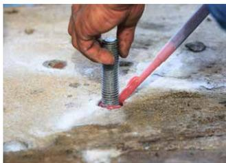
Figure 2: Epoxy Anchor
