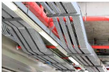
Figure 1: Threaded Rod as Hangers
