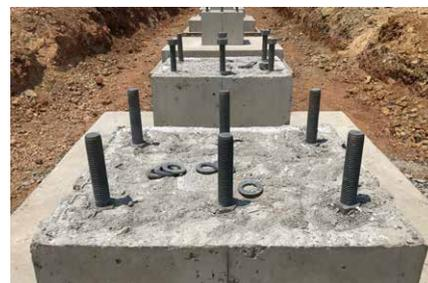
Figure 5: Anchor Bolts for Building Column
